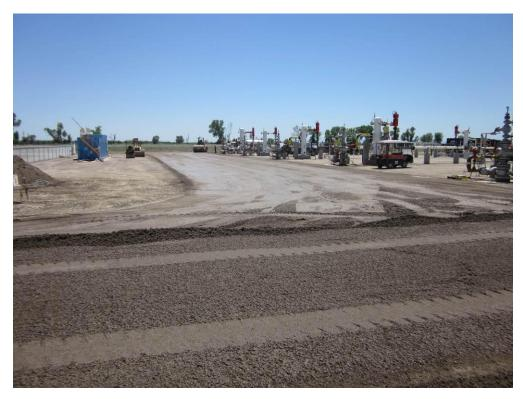
**Photo 1:** The Remote Well Pad site has been graded and installation/rolling of final base material was underway.
