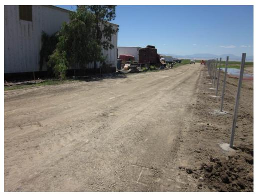
**Photo 4:** The silt fence along the southern boundary of the Compressor Station site is in need of repair or removal, based on recommendations by the project QSP responsible for implementing the SWPPP.
